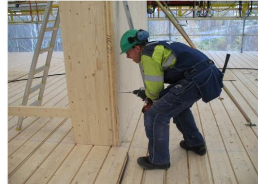
Ensure screws are driven in the side grain!!
