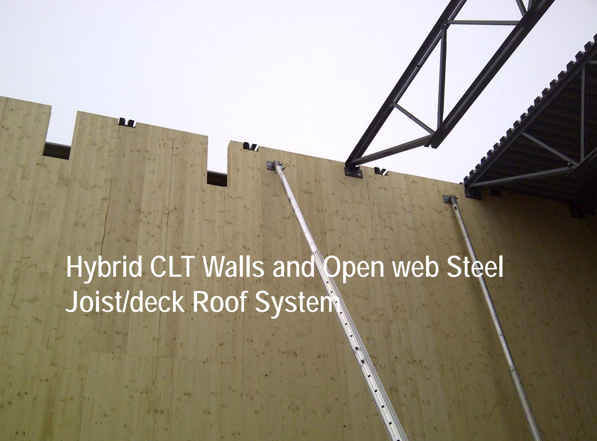
A photograph showing the construction of a hybrid structure. The walls are made of light-colored cross-laminated timber (CLT) panels. The roof is an open web steel joist/deck system. Two long, silver metal poles are leaning against the CLT wall. The sky is overcast and grey.
