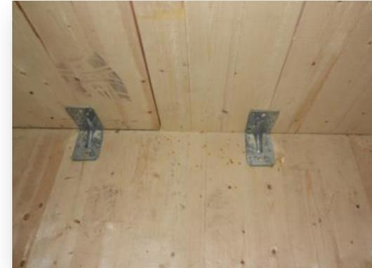
Most commonly used connection system in CLT assemblies in Europe & Canada
