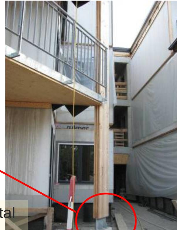
CLT panel/post to concrete pedestal through metal brackets and internal metal plates
