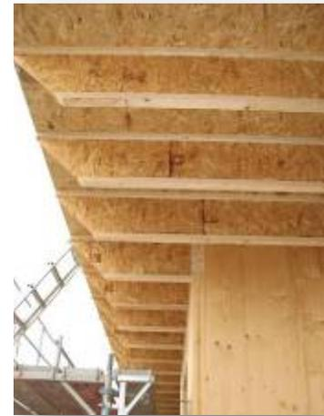
CLT Wall & I-joisted floor with EWP rim board and blocking. Self tapping screws are used
