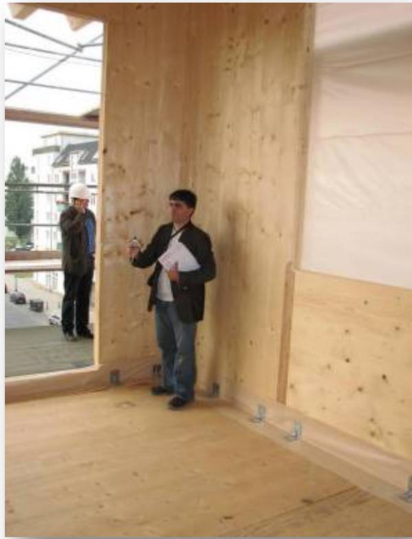
1<sup>st</sup> storey wall to floor/roof → self tapping screws
