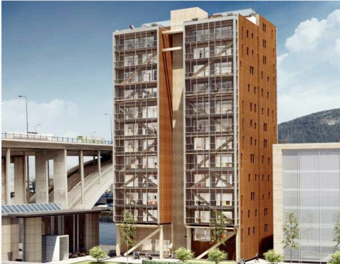
14-storey, Bergen, Norway (2014-15)
