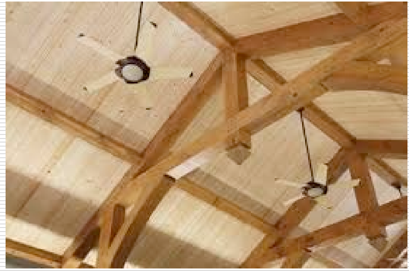
Massive timber – slower or no burn-through
