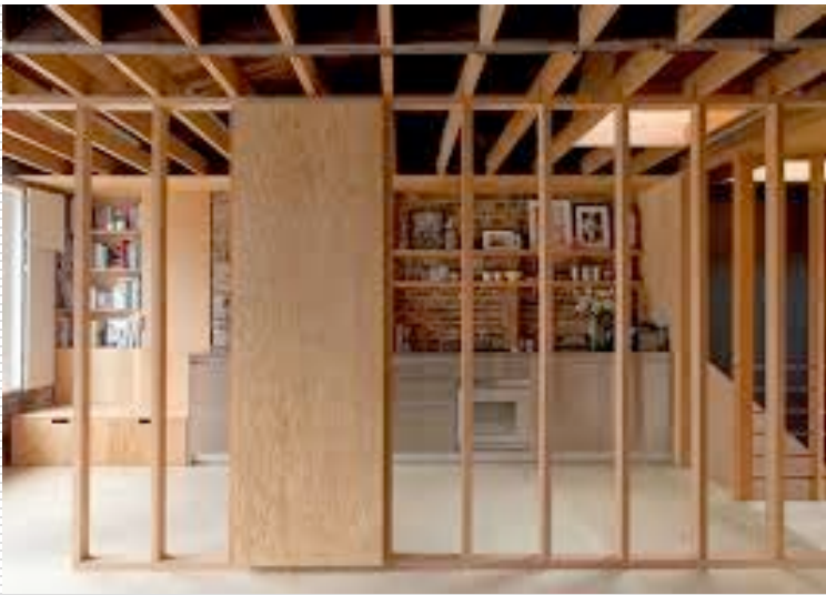
Light framing – faster burn-through
