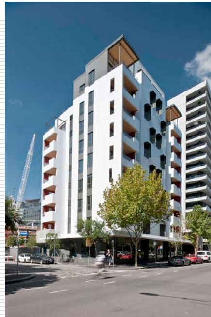
10-storey CLT building, Melbourne
