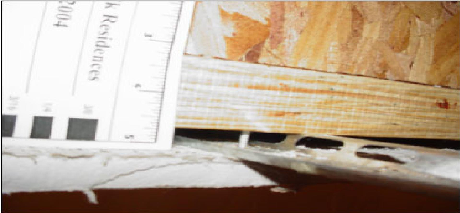
*This photograph shows where the builder has used excessively long screws to fasten the gypsum ceiling. This results in the resilient channel being anchored to the wood joist eliminating the vibration and sound isolation provided by resilient channels.*
