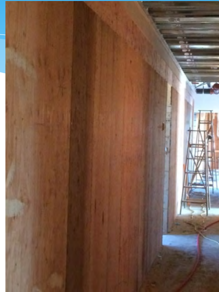
• Corridor and demising walls are shear panel walls
