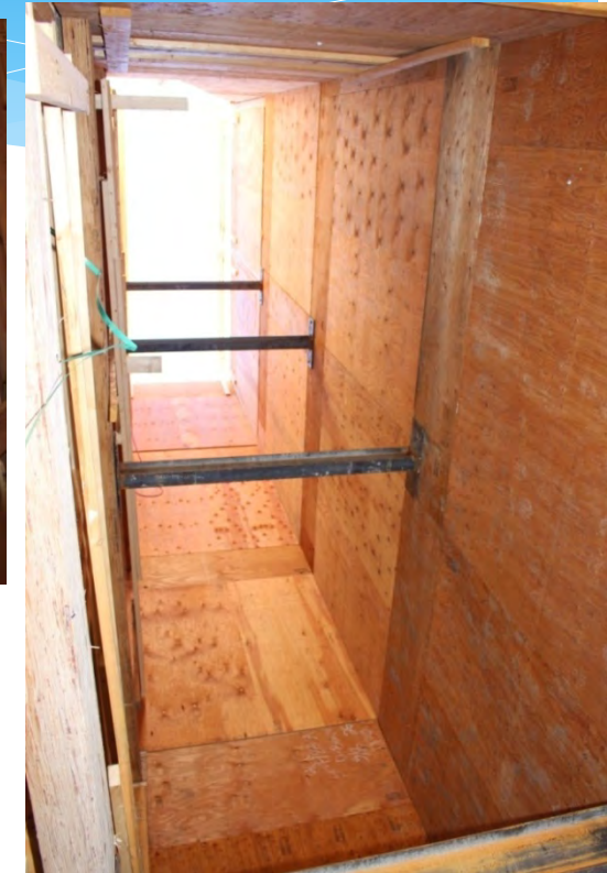
Plywood lined interior
