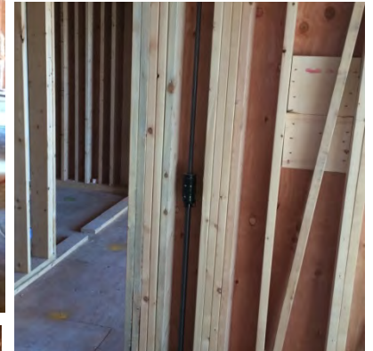
• Solid Wood built up timber sections within walls
