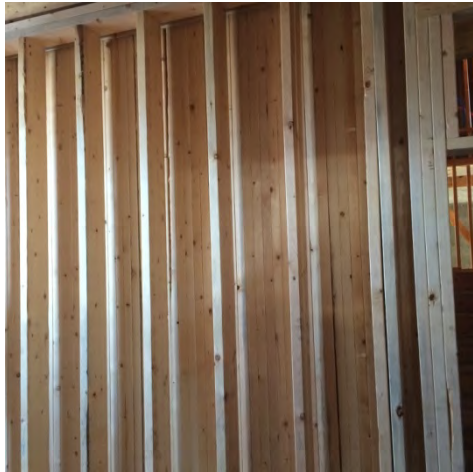
• Close Stud Spacing typical at lower floors
