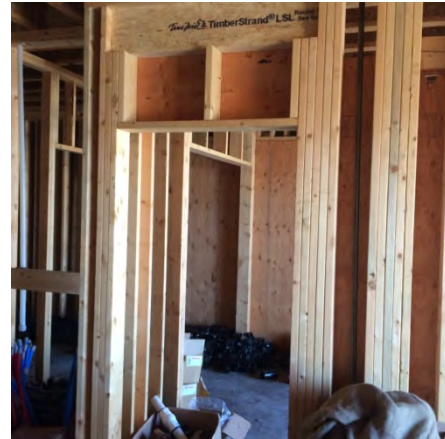
• Solid Wood built up timber sections within walls
