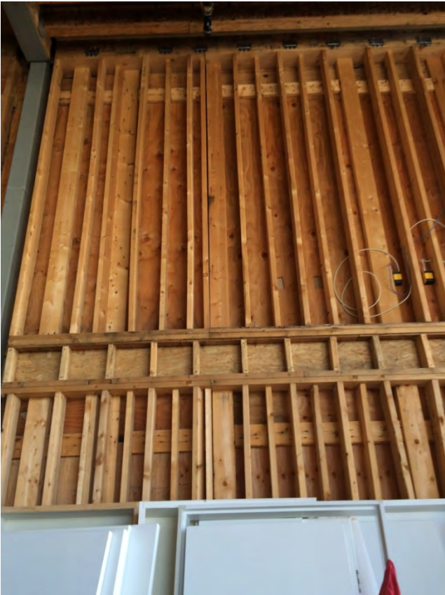
Installed smaller cavity spaces and ceiling spaces
