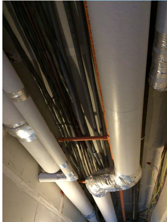
Systems running in non-combustible concealed space above corridor
